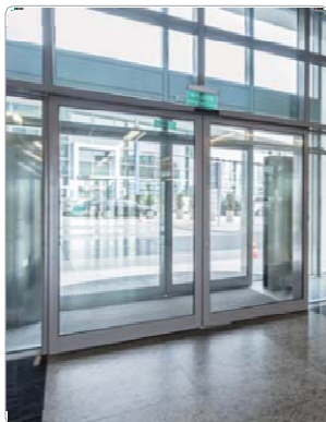
Entrance door in building 건물출입문
